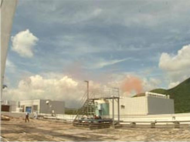
plume rise allows much better dispersion, and is expected to significantly reduce the rooftop chemical concentration. On the other hand, the short stack height allows us to retain the aesthetic outlook of the Laboratory Block.
